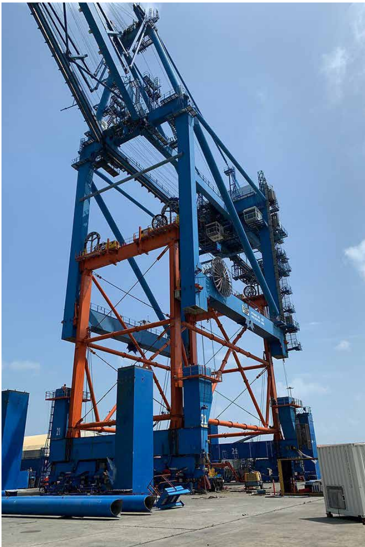
LEFT The lifting frame deployed with custom design and fabricated pieces ready for installation
