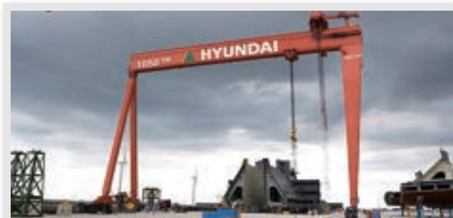
▲ 1650T Capacity Goliath Gantry Crane
