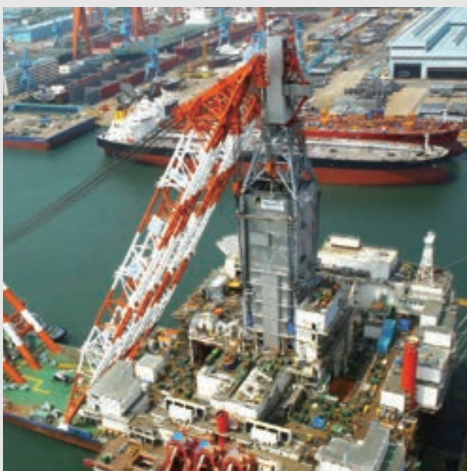
▲Derrick for Semi-Submersible Drilling Rig
