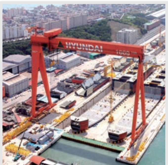
▲ 1600T Capacity Goliath Gantry Crane
