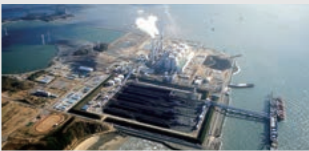
▲ Coal Handling System
