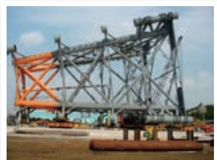
▲ Mega Steel Structure
