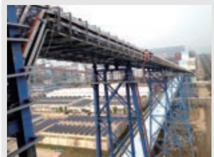
▲ Conveyor Belt System
