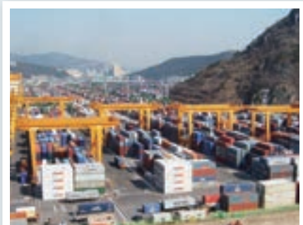
▲ Automated Transfer Crane for Busan Port
