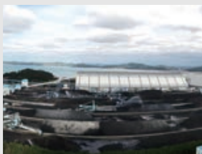
▲ Coal Storage Facility (Shed Type)
