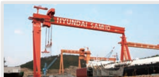
▲ 900T Capacity Goliath Gantry Crane
