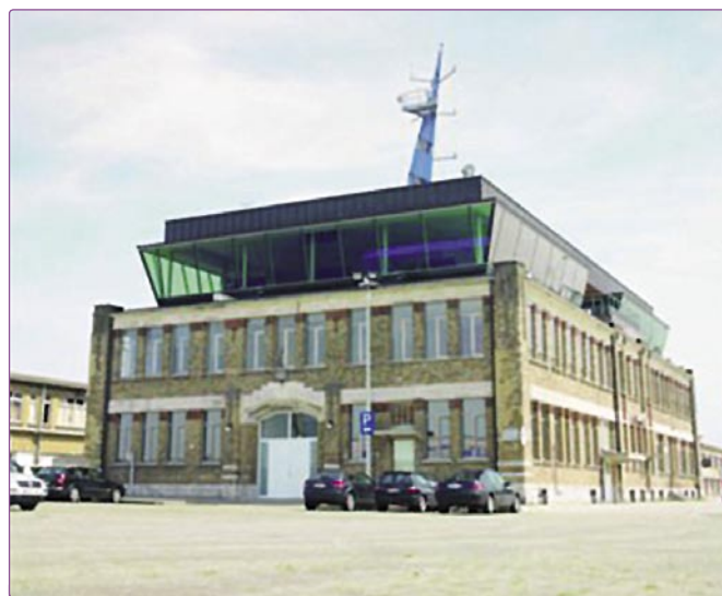
The new MRCC, Ostend.
