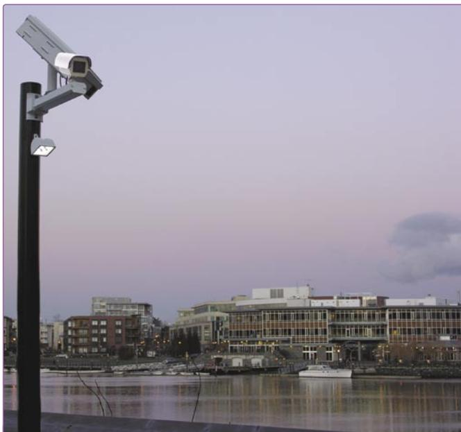
Solar-powered floodlight and security camera installed in inner-harbour, Victoria, BC, Canada.
