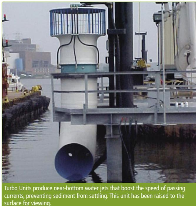
Turbo Units produce near-bottom water jets that boost the speed of passing currents, preventing sediment from settling. This unit has been raised to the surface for viewing.
